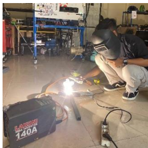
Figure 5. Welding Process of the Steel Frame
